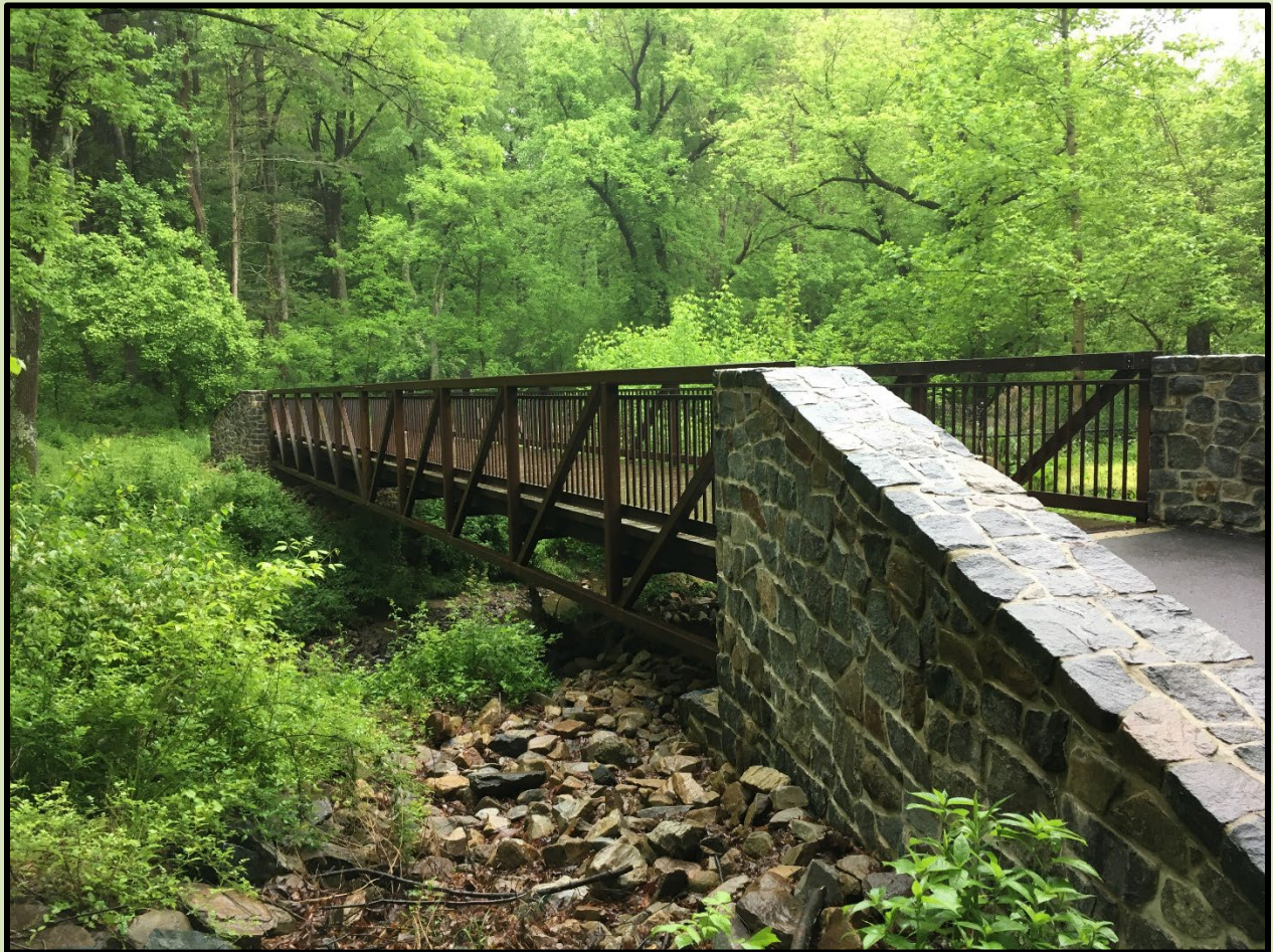
New Rocky Run Bridge
