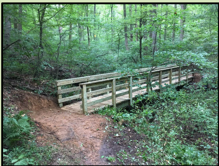
Typical Trail Bridge
