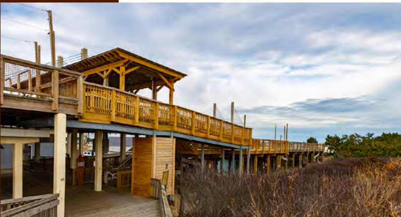
Big Chill Beach Club ramp at Delaware Seashore State Park
