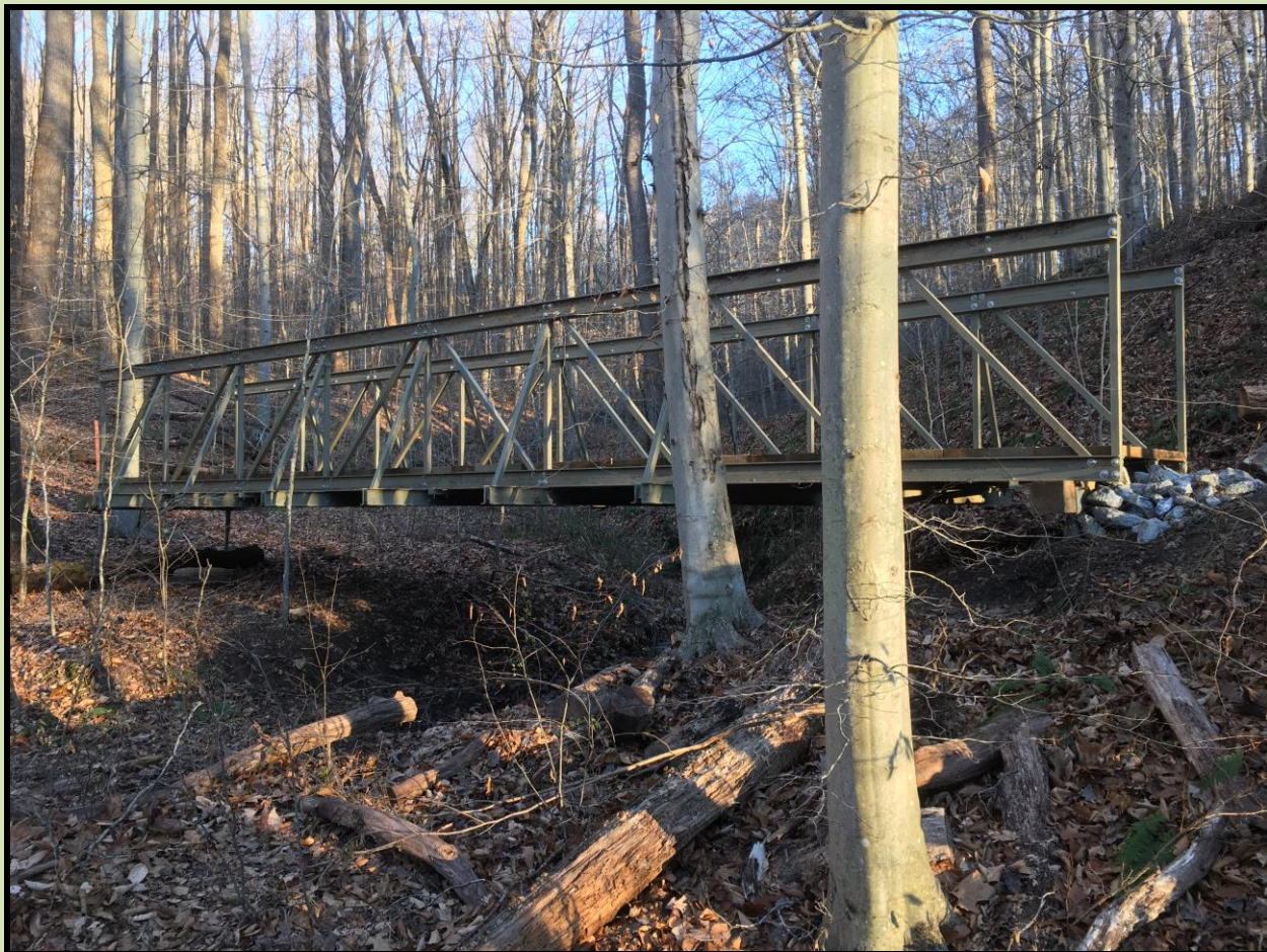
New Bridge on the Charles Bailey Trail
