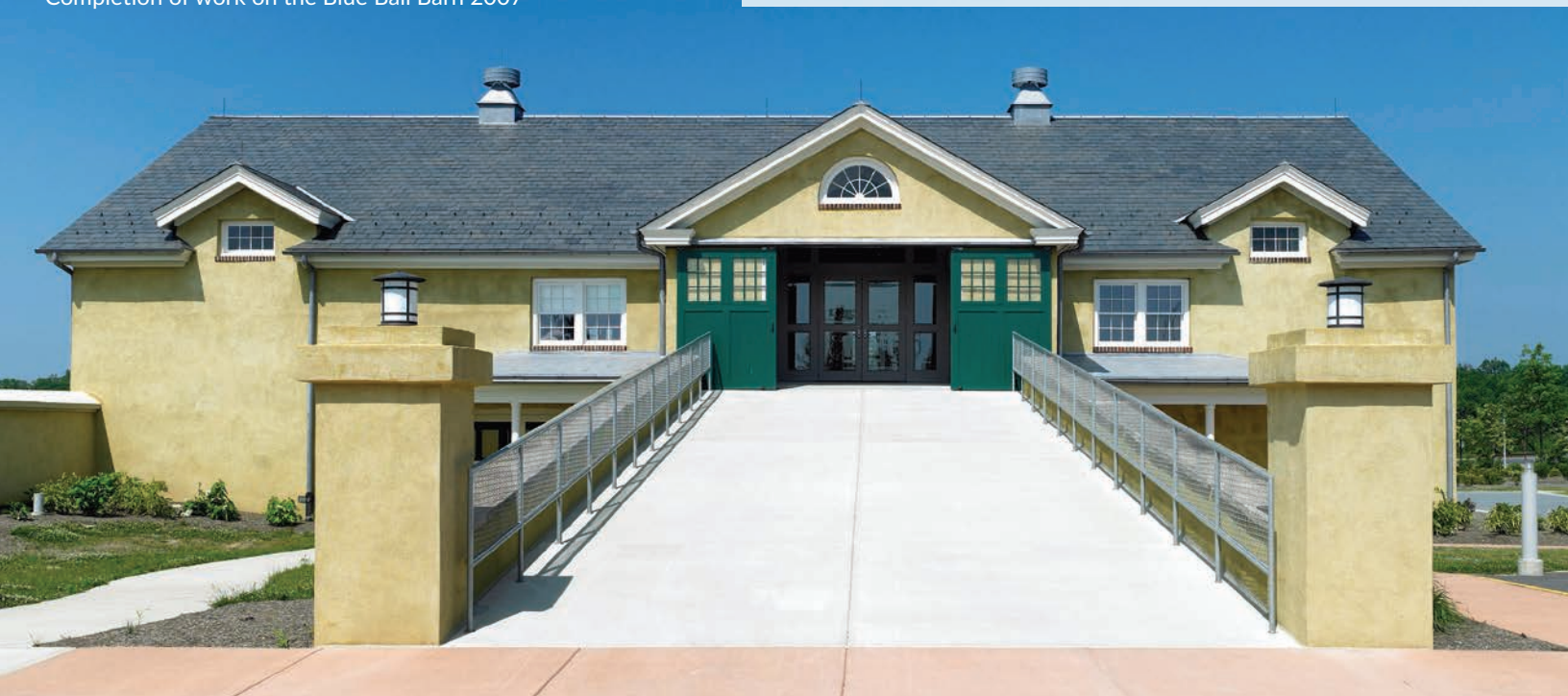
Completion of work on the Blue Ball Barn 2007
