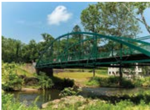
Bridge at Auburn Valley State Park
