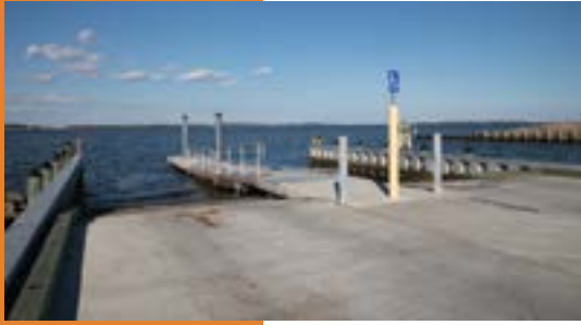
Boat Ramp at Indian River Marina
