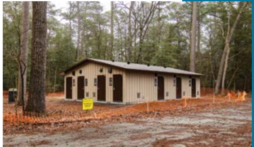
Bathhouse at Trap Pond State Park
