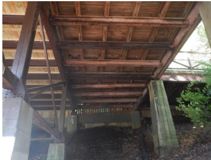
Photos 5: Series of short spans on North side of the bridge
