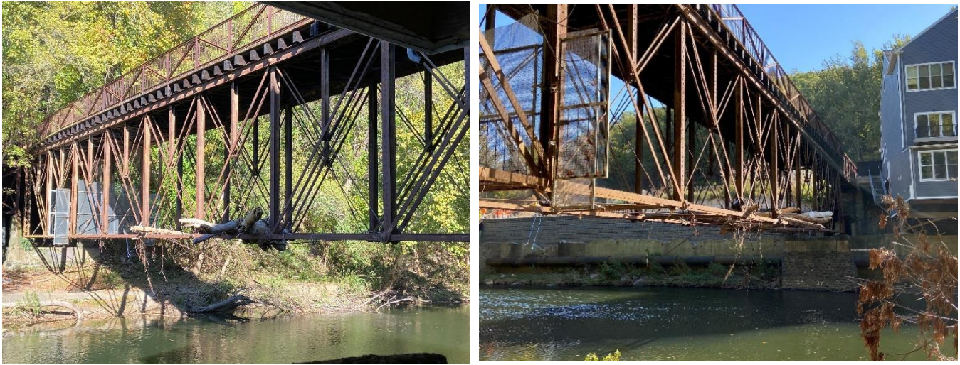
Photos 3 and 4: Main deck truss bridge
